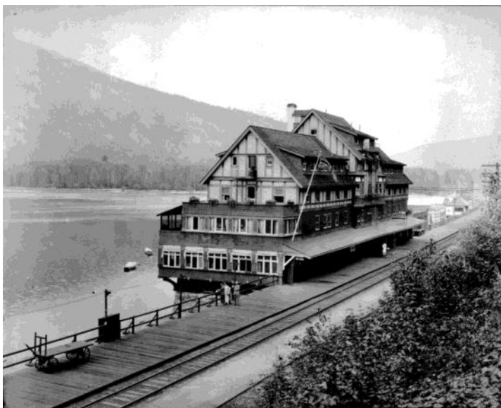
Fig. 1. View facing east of the CPR's Sicamous Hotel and depot, c. 1920. Photo from Canadian Pacific Archives. Downloaded from the Shuswap Passion website
