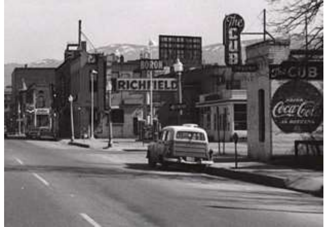
The subject of this project is visible on the far right. At one time, it operated as The Cub Tavern from 1948 until the late
