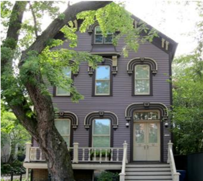
Fig. 3. This is a balloon frame house in Chicago, built circa 1870. The window above the door was a stairwell light to the upper level, as evidenced by the smaller space between the window sill and the door's transom light. There was no floor below, thus allowing for the transom light and taller trim over the door. The overall size of the window is the same as the other second floor windows. For the sake of the second floor symmetry, the window is not centered over the door.
