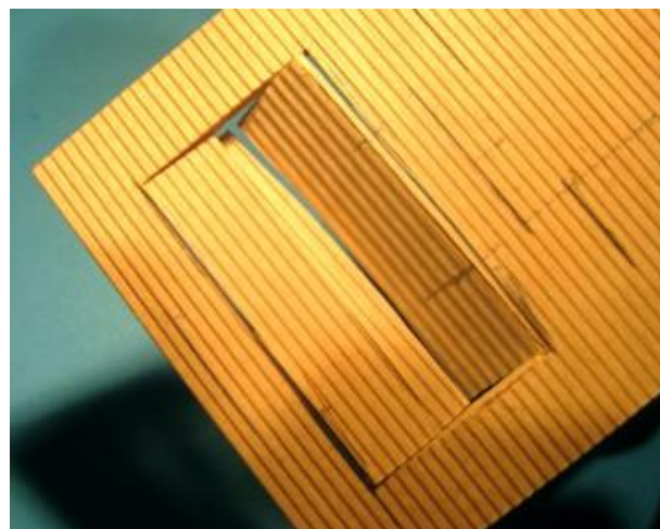
Fig. 10. The two final cuts in a window or door opening showing how they can help remove the waste material.
