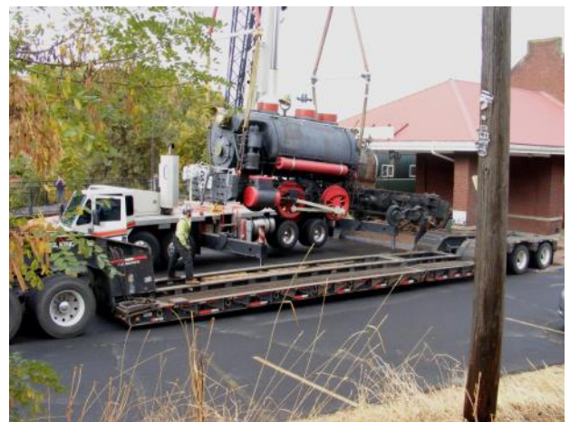
Lifting and loading locomotive
