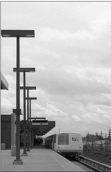
1972 - BART station, Richmond, CA
