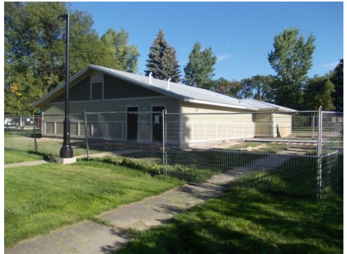
Interior and Exterior views of the SAMRC club building expansion in Gyro Park. (Photos by Doug Wingfield)
