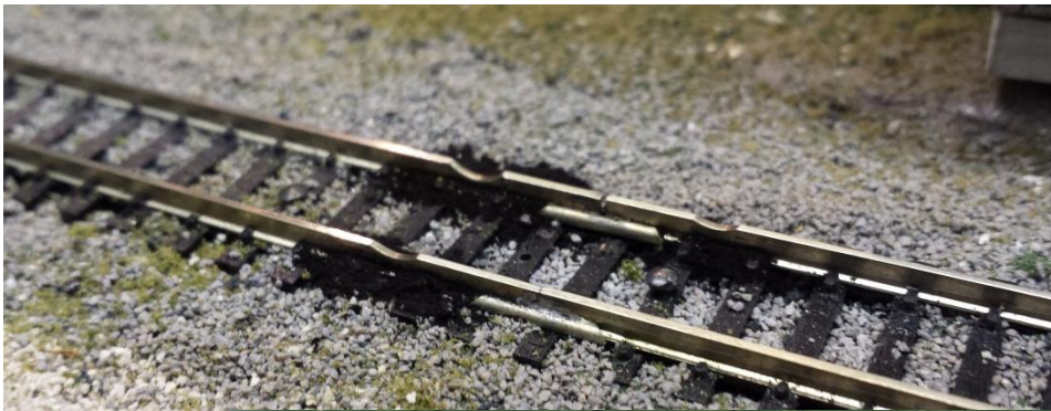
Left – The damaged track.
